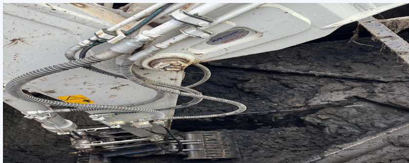
Specialist grab attachment clearing between silo strengthening supports
