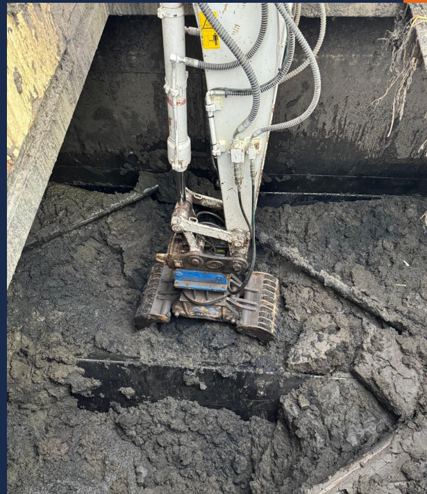
Inside the cake silo during dig-out operations
