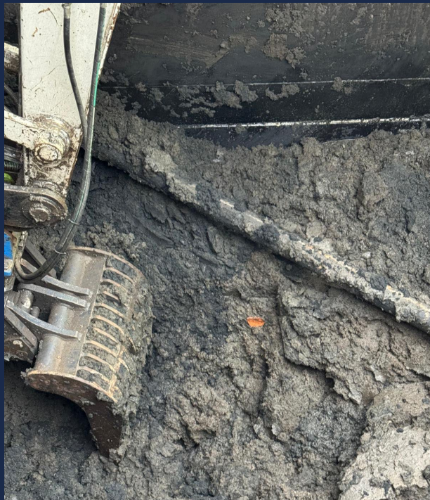
Specialist grab clearing cake from silo chamber
