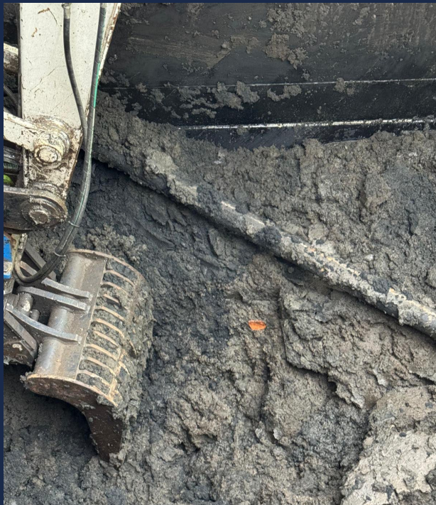
Esholt WWTW site - overnight mobilisation
