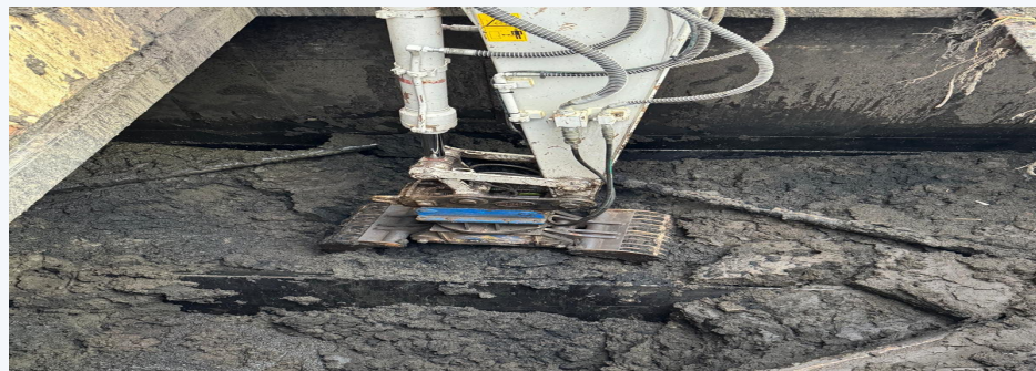
Deep access within the cake silo screw shaft chambers, Esholt WWTW
