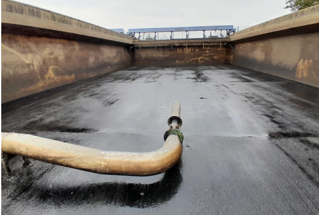
Interior view of cleaned storm tank
