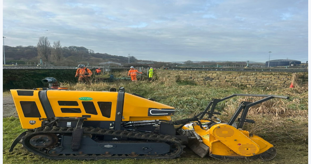
Tracked Mulcher – Bankside & Perimeter Clearance
