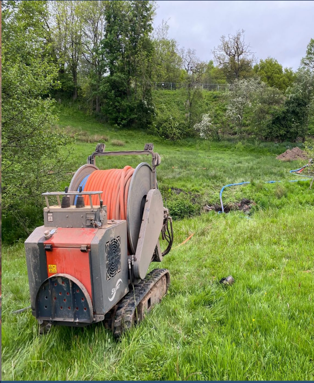
MRMS mobilisation to breach location
