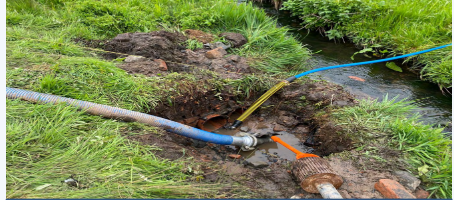
De-watering setup at culvert outlet with twin pipe connection
