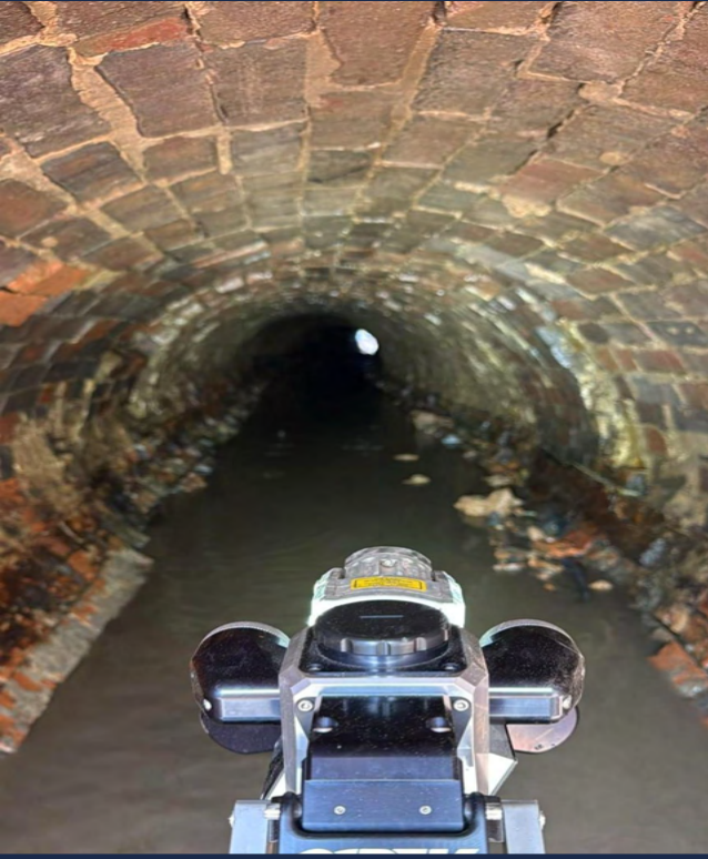
Silent reel unit - remote deployment in field
