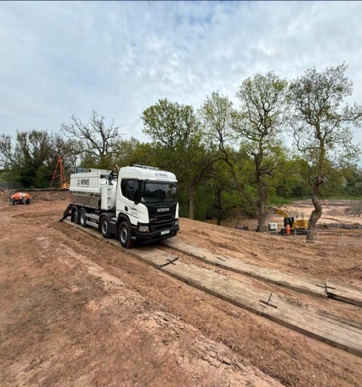
Excavated culvert inlet - breach site
