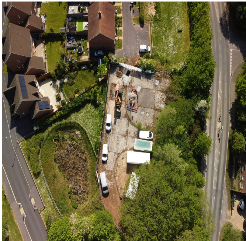
Chamber construction & connection works — Bramley Storm Tank
