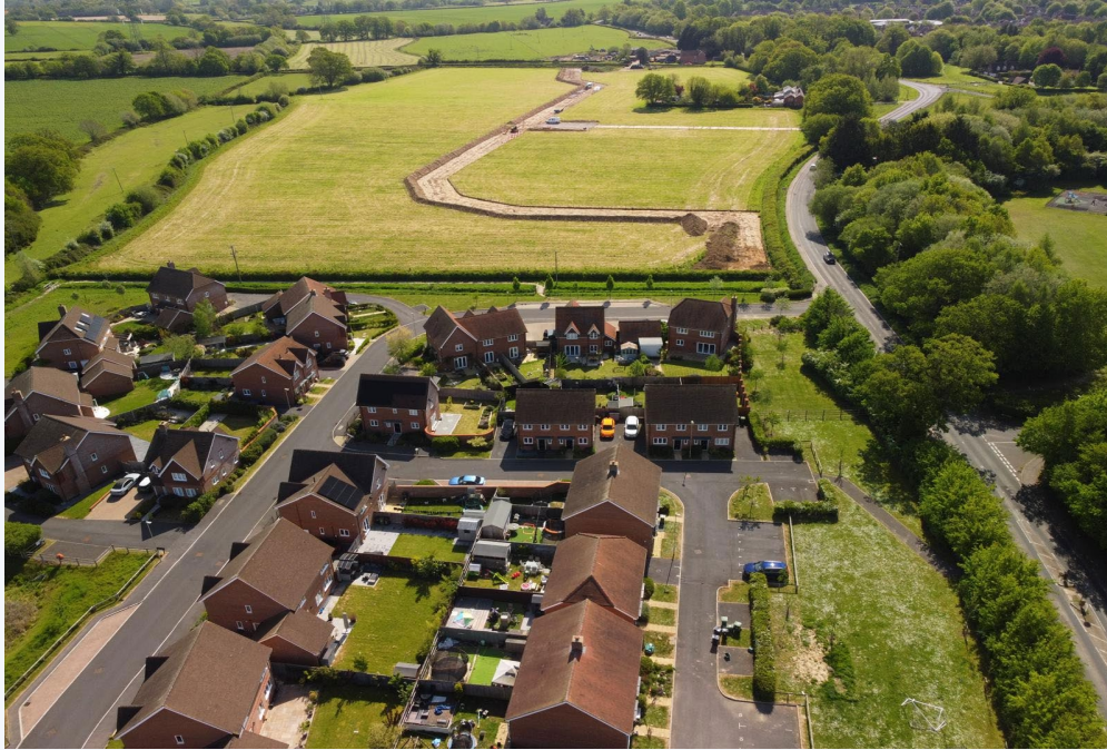
Aerial view of the Bramley Sewer Scheme route
