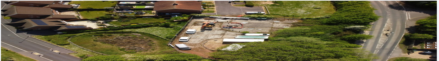
Compound & chamber construction works — Bramley Storm Tank connection
