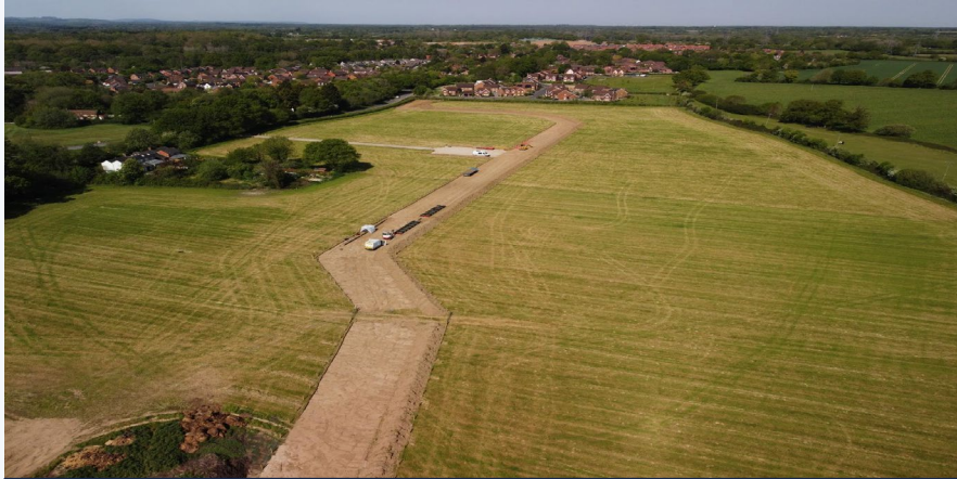
Easement — topsoil strip & haul route
